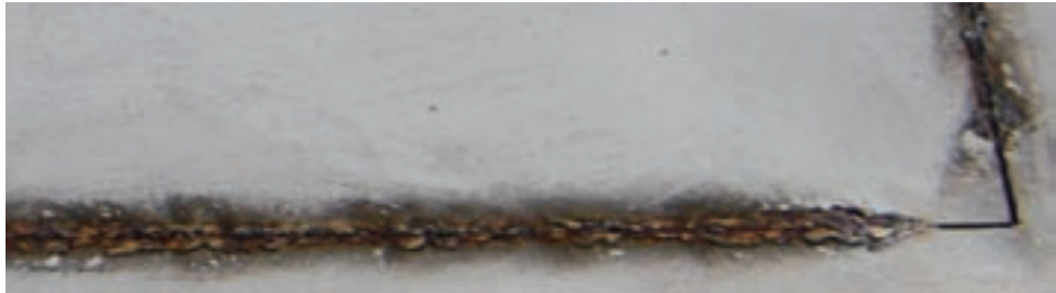
Improper cut example
